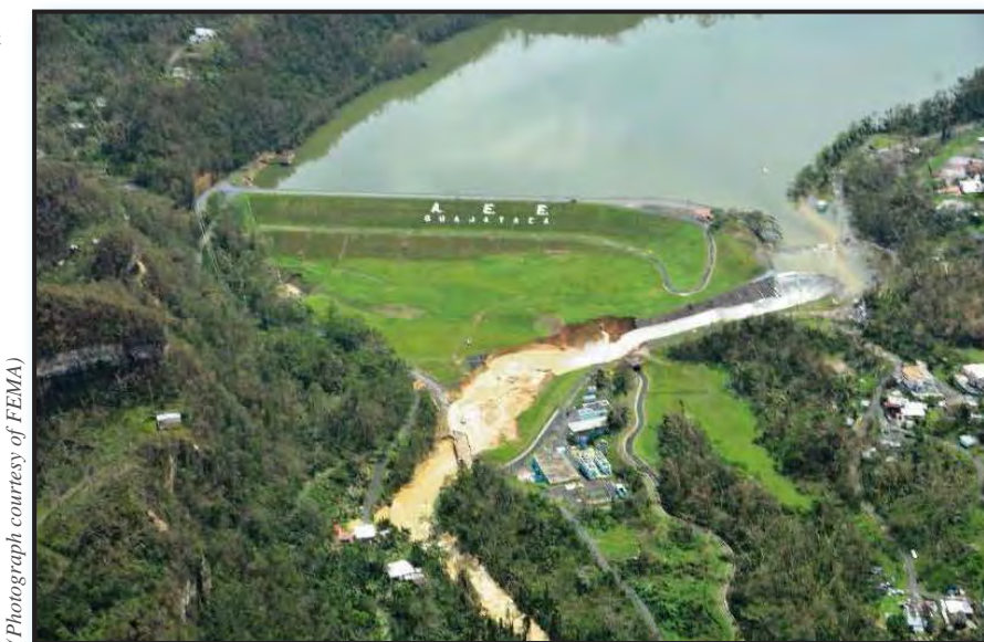
Guajataca Dam in Puerto Rico
