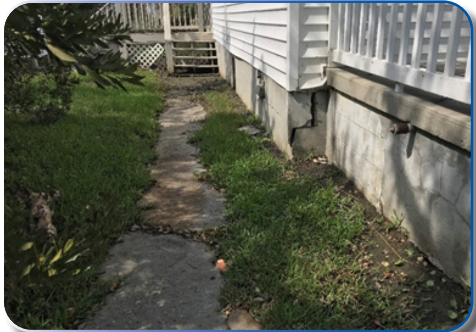
Foundation Damage on Ocracoke as a Result of Hydrostatic Force
