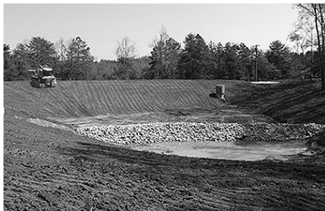
Retention Pond Under Construction
